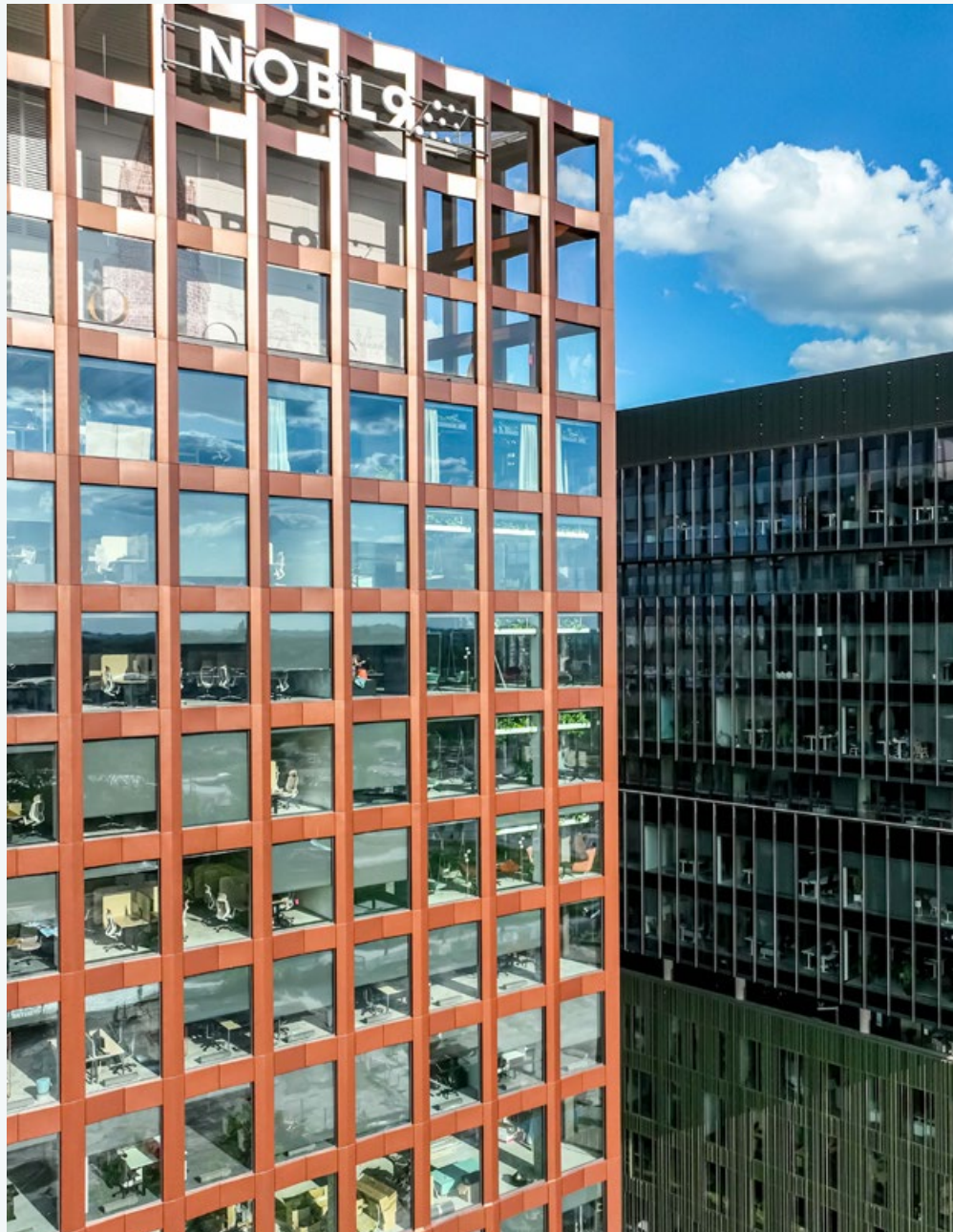
The rust-red Nowy Rynek E property towers over the green-coloured Nowy Rynek D in Poznan. Both properties feature large glass sections that allow plenty of daylight.
