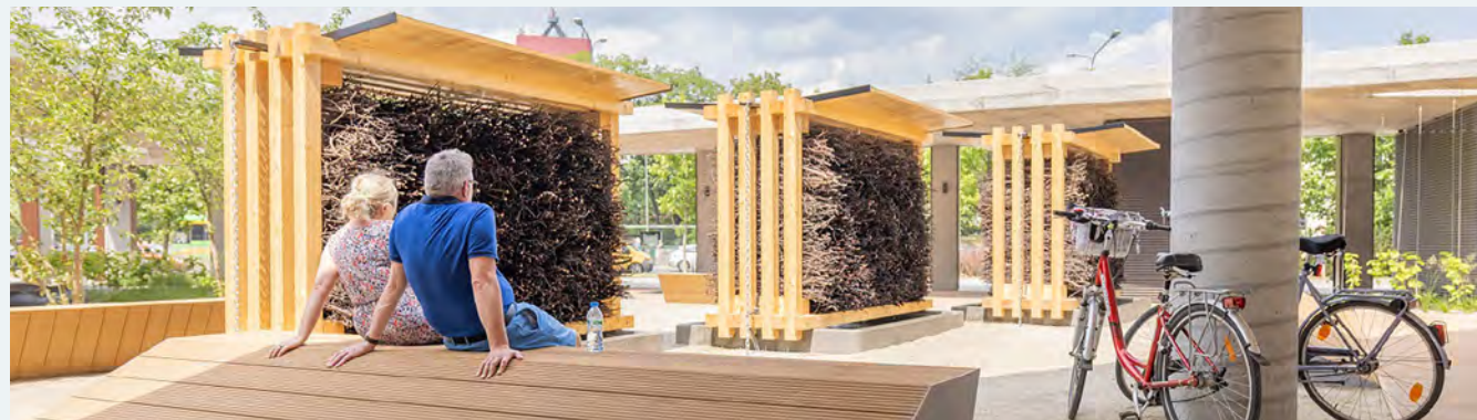
Outside of the Nowy Rynek properties, there is a square with park benches and gravel pathways. These installations are designed to enhance air quality and create a microclimate offering health benefits similar to that of fresh sea air.
